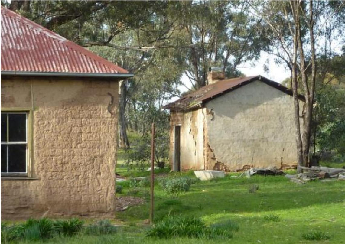
Figure 3 Former Kelly farm house, Caldow Road, Woodvale (W8). The mud brick structures were erected in the early twentieth century.
