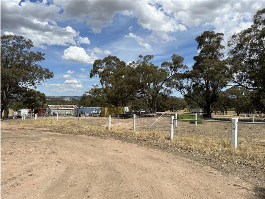
Figure 6: View facing the structures on site looking east from the end of Hunt Road.
